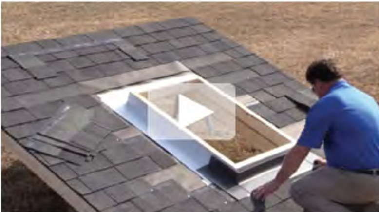
VELUX Install Video: Replacing Curb-Mount Skylights
