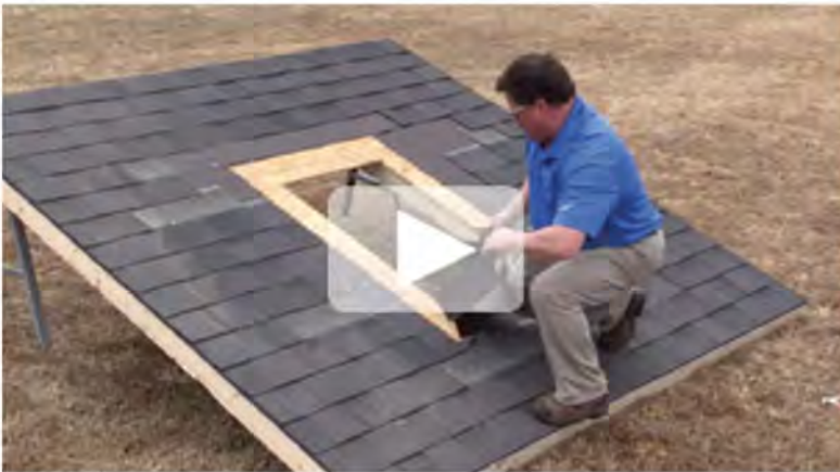
VELUX Install Video: Replacing Deck-Mount Skylights
